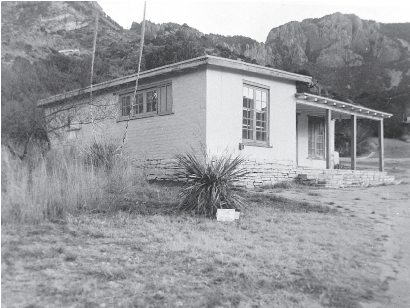
Figure 4: Chisos Basin Store, Big Bend National Park, Texas. Perspective view from Northwest Corner. From Library of Congress, Washington D.C., HABS TX-3399-2.
