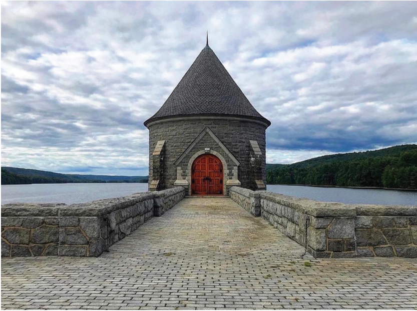
Figure 5: Saville Dam, Barkhamsted, Connecticut. Photo by Joseph Fortuna.
